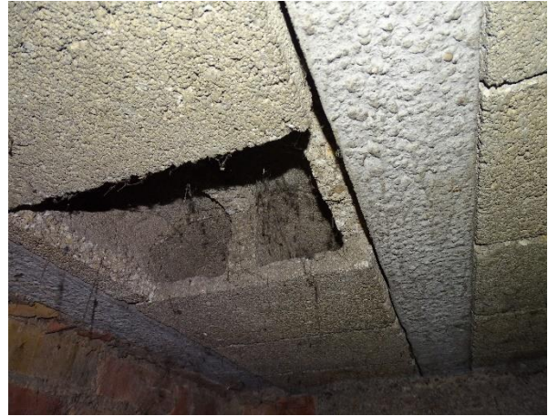
Abb. 8: Offener Hohlblockstein in Kellerdecke
